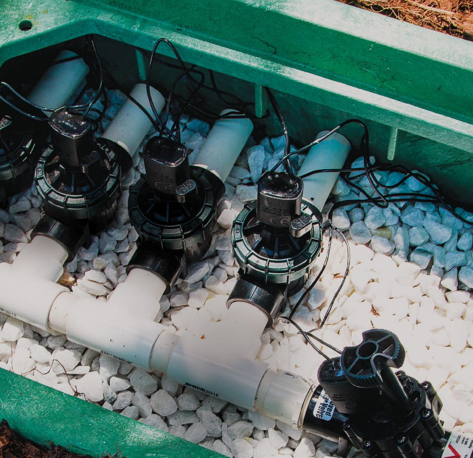
**The Holman and K-Rain range of solenoid valves are made from high quality UV resistant PVC construction.**
