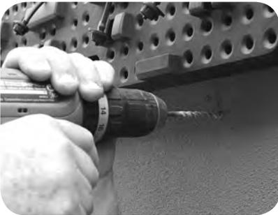
4) If attaching to a solid wall such as brick or concrete, use a 6.5mm masonry bit to drill all three holes.
