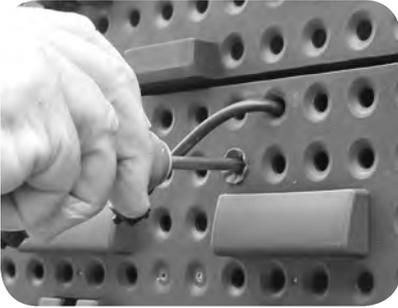
Next you need to mark the wall to position the stainless steel holding bracket.
