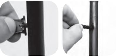
e) Use the 4mm punch to punch a hole in the poly pipe. Insert the joiner connected to the tube.
